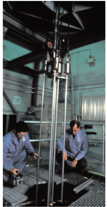
Coolant Water Filtration at a Nuclear Plant
