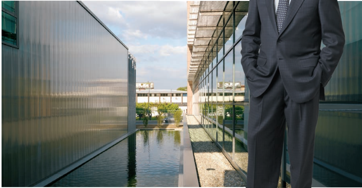
Pall's new facility in Buccinasco, Italy incorporates the latest in green technologies to protect the environment and lower operating costs.
